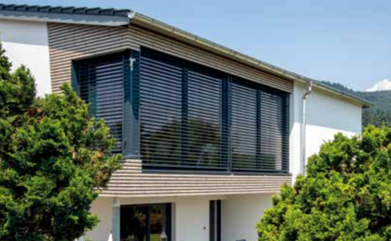
Exterior and facades
